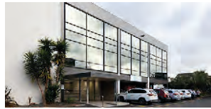
308 Great South Road, Greenlane
