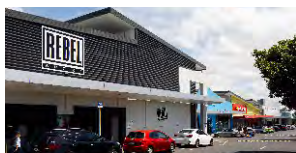
Albany Mega Centre and 11 Coliseum Drive, Albany
