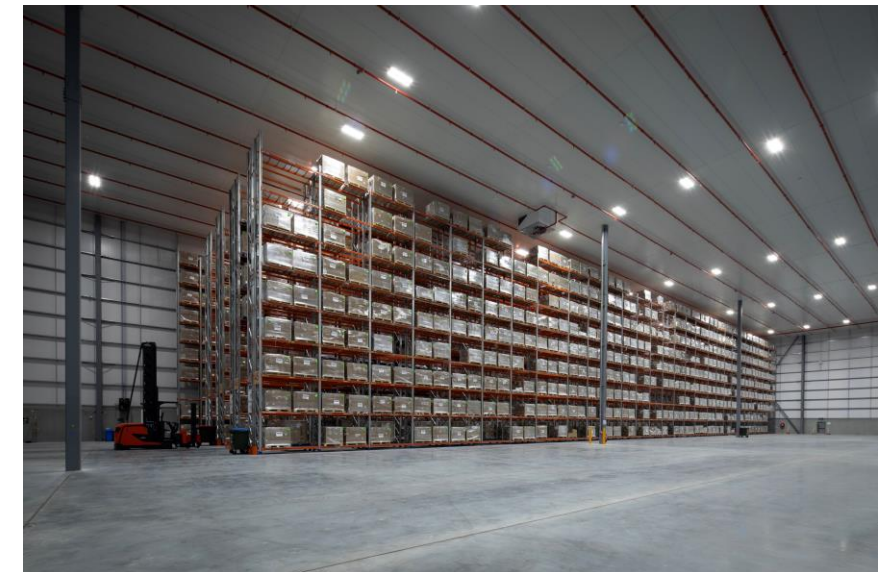
New Contract Logistics DC, Sydney.
