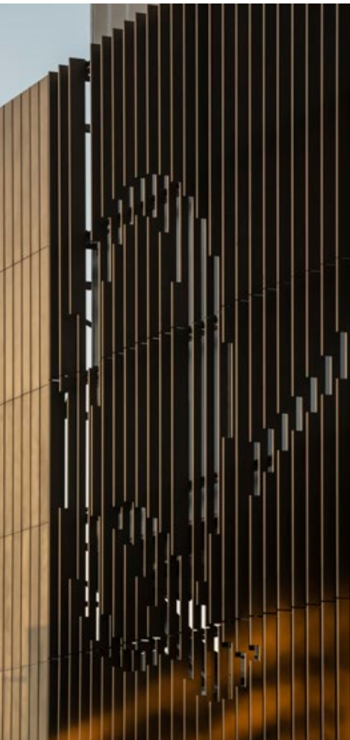
Queensgate Shopping Centre, Wellington
