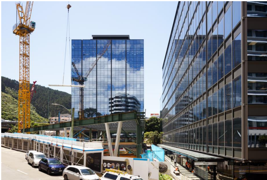
Construction of 40 & 44 Bowen Street
