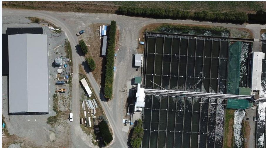
Tentburn Hatchery – aerial view
