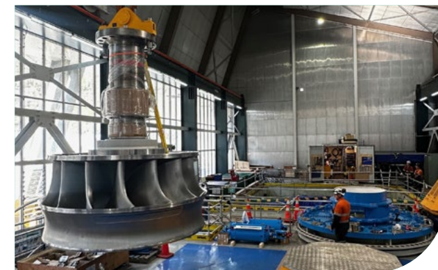
New turbine being installed at Matahina
