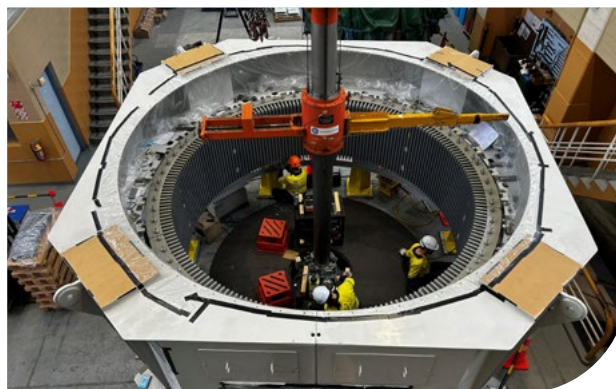
New Highbank generator under construction
