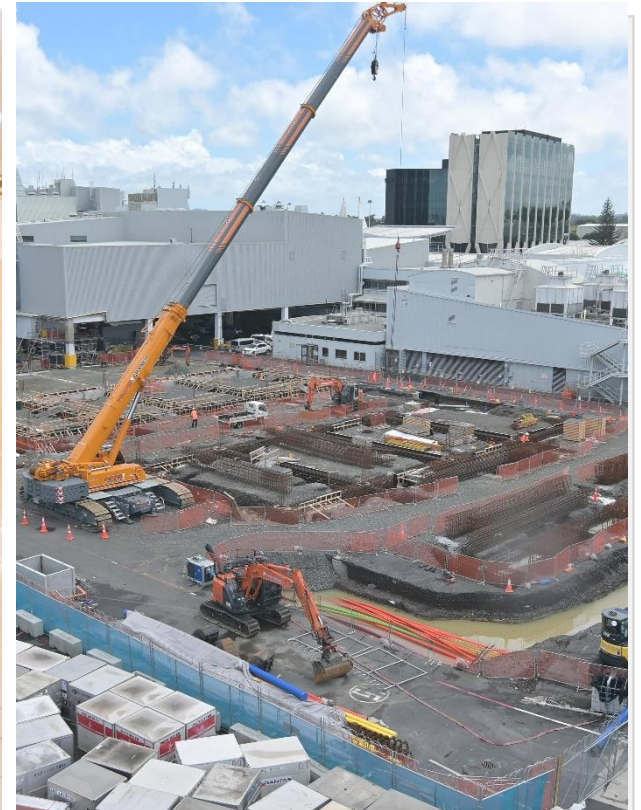
Foundation work on the Eastern Bag Hall
