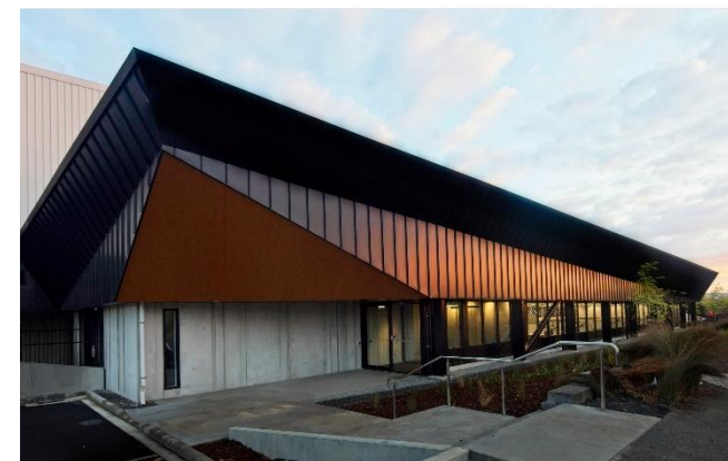
New temperature-controlled office and warehouse development at 6-8 Kapua Drive
