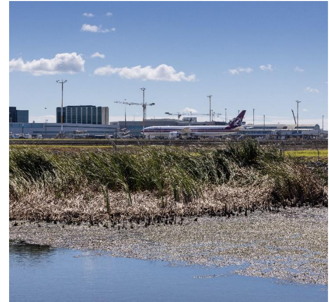
Airside stormwater pond
