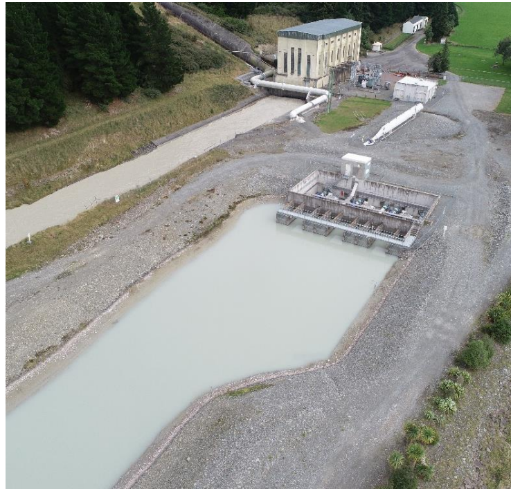
Irrigation pumps at Highbank Scheme
