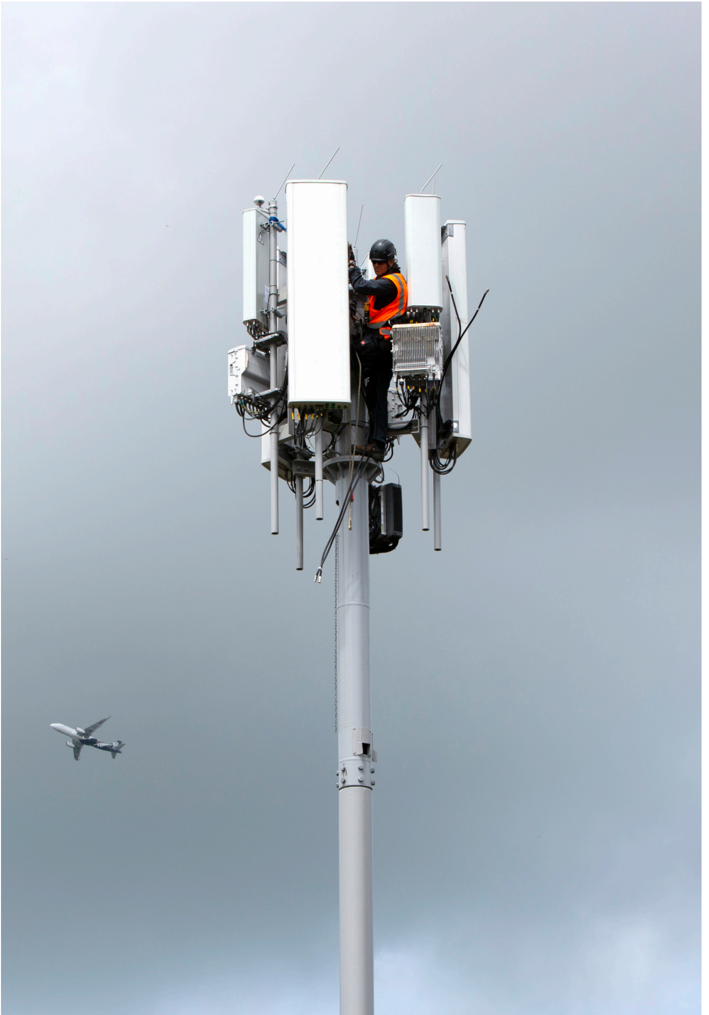
Vodafone 5G tower installation, Māngere, Auckland
