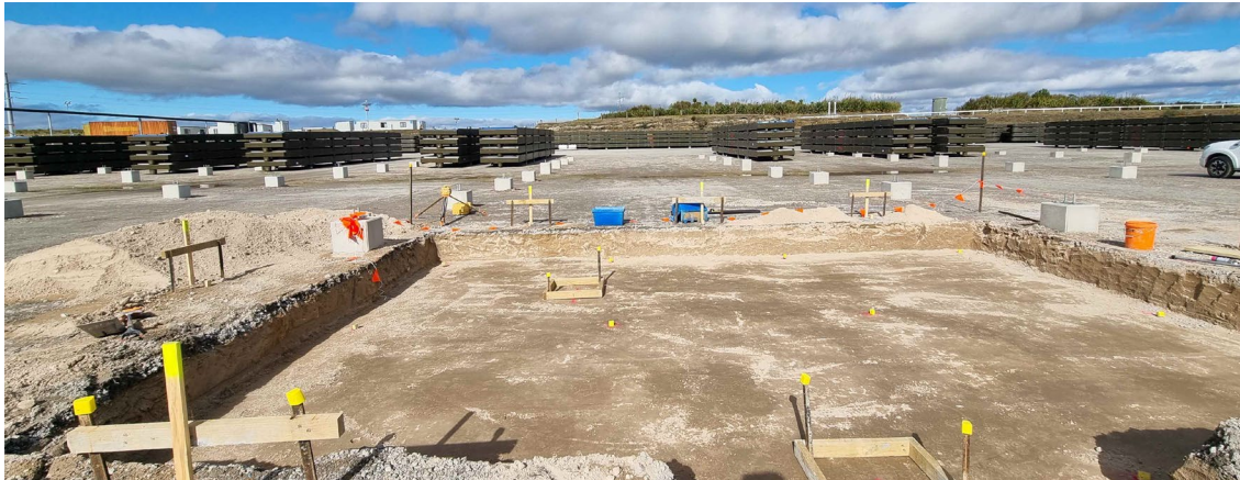
Ngā Tamariki OEC5 under construction
