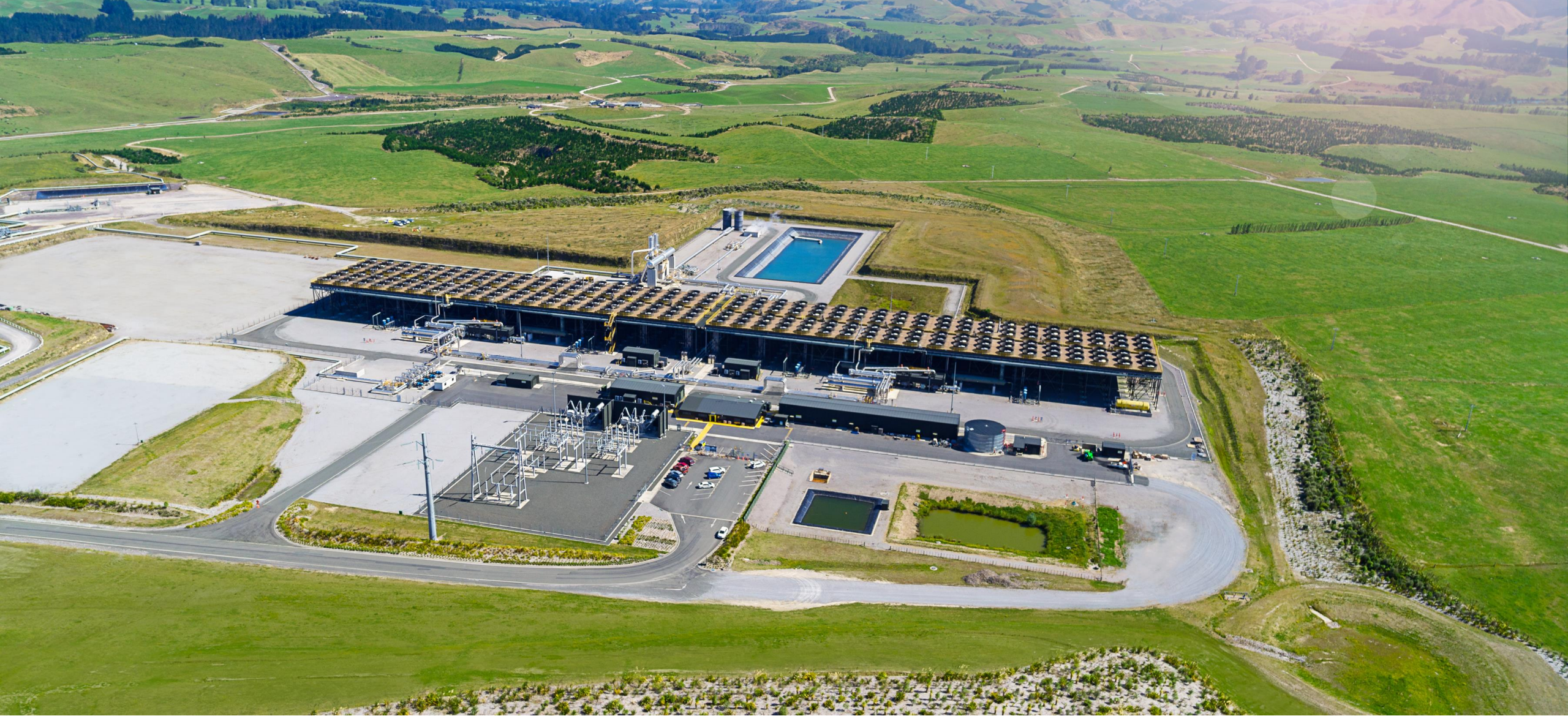
Ngā Tamariki geothermal station
