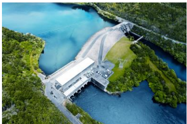
Waipāpa (1961) 51MW 235GWh
