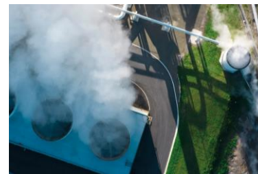
Kawerau (2008) 106MW 875GWh
