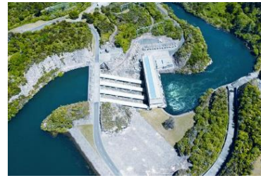
Ōhakuri (1961) 112MW 405GWh
