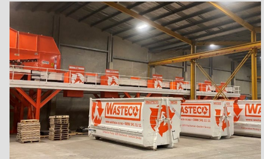
3,600m 2 Sorting facility in Christchurch
