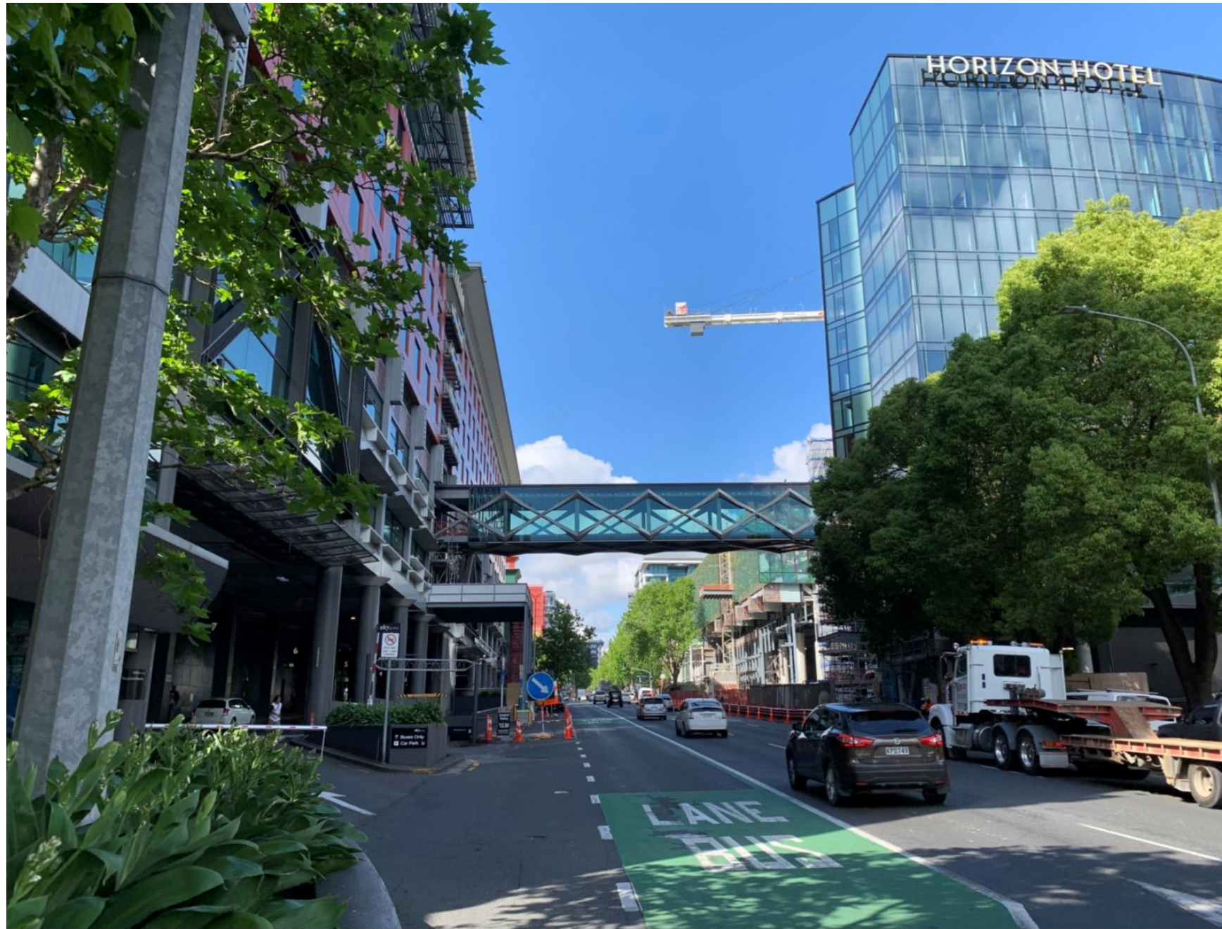
View from Hobson St – new linkway bridge
