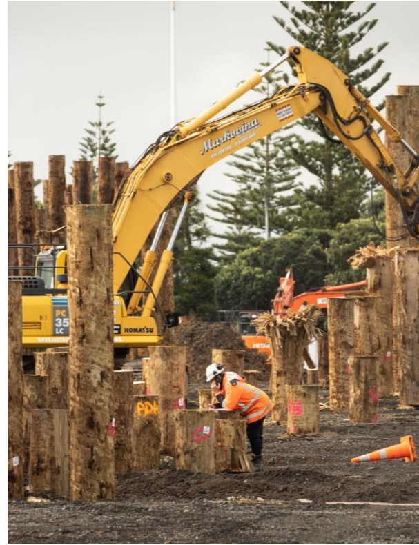
Foundation piles for the Transport Hub
