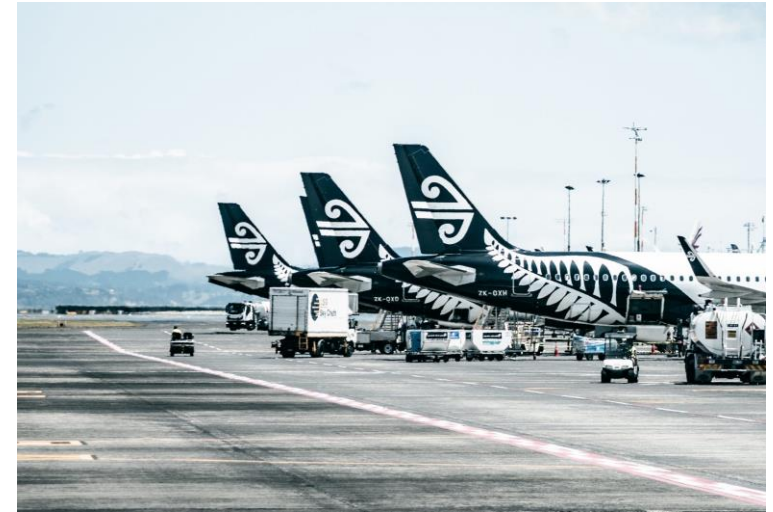
Auckland Airport airfield
