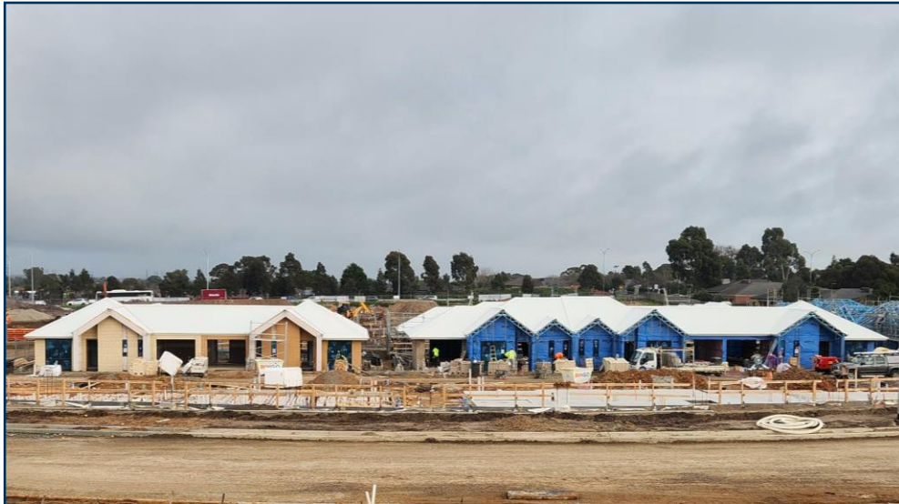
Site progress - Summerset Cranbourne North (Melbourne)
