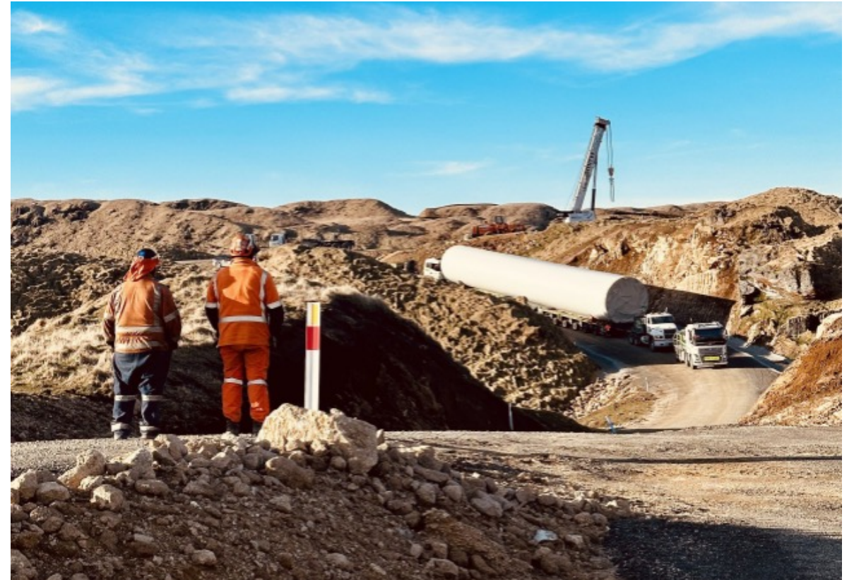
Turbine tower section being transported at Meridian's Harapaki wind farm
