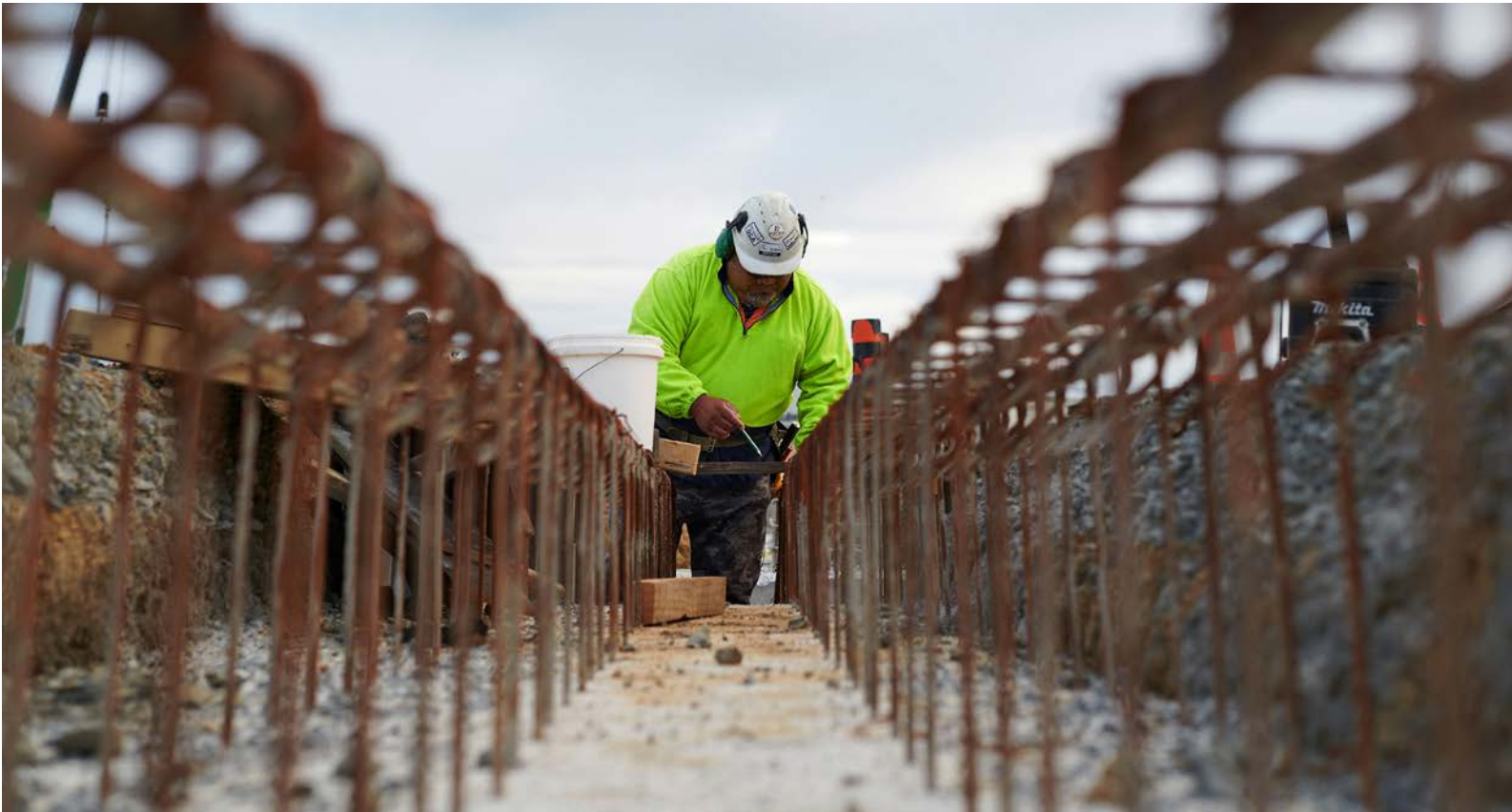
Riverside Warehouses under construction, Highbrook Business Park
