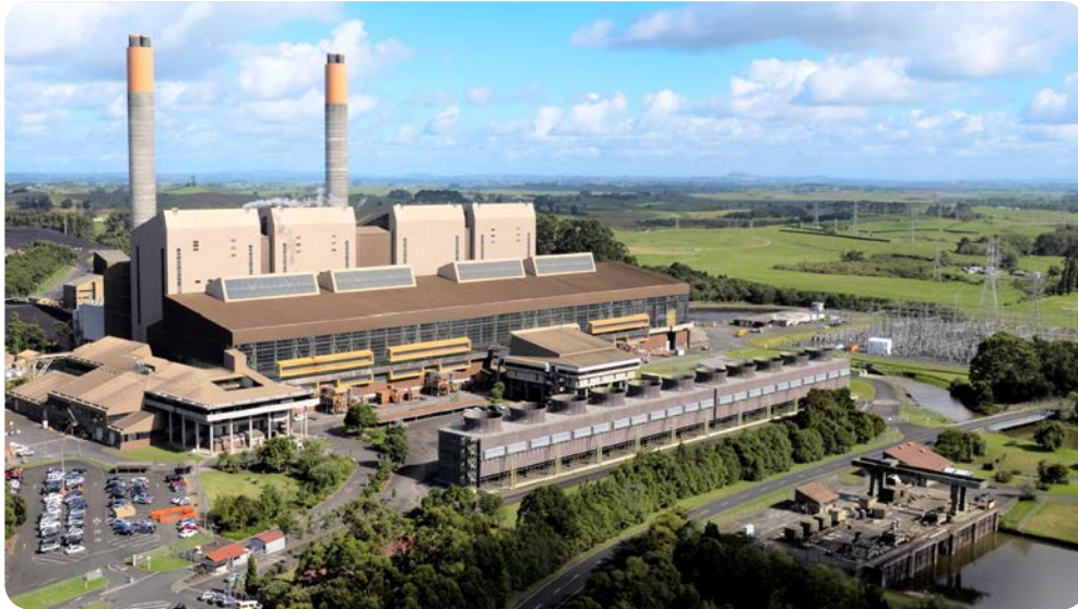
Huntly Power Station
