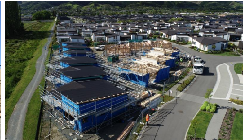
Waimea Plains, Richmond | 26 villas Delivery over 2H
