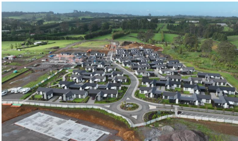
Te Puna Wairoa, Kerikeri – 281 units (on completion) 53 units delivered; 228 units to be built
