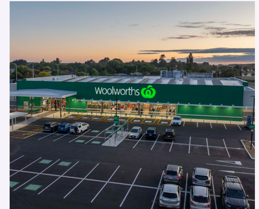
New Woolworths supermarket at Waimakariri Junction, created for Investore – delivered on time and within budget, achieved a 5 Green Star Design rating and targeting a 5 Green Star As Built rating. This property has been leased to Woolworths for an initial term of 12 years, and a total term of 35 years if all rights of renewal are exercised. The development will deliver a yield on cost of 5.5% (including land).
