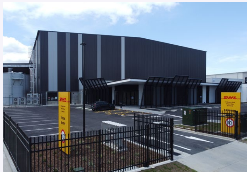
New industrial development at 34 Airpark Drive, Auckland – delivered on time and within budget for Indstre, and targeting a 5 Green Star As Built rating. This property was leased on completion to DHL for a 10 year term, and delivers a yield on cost of 5.8% (including land).
