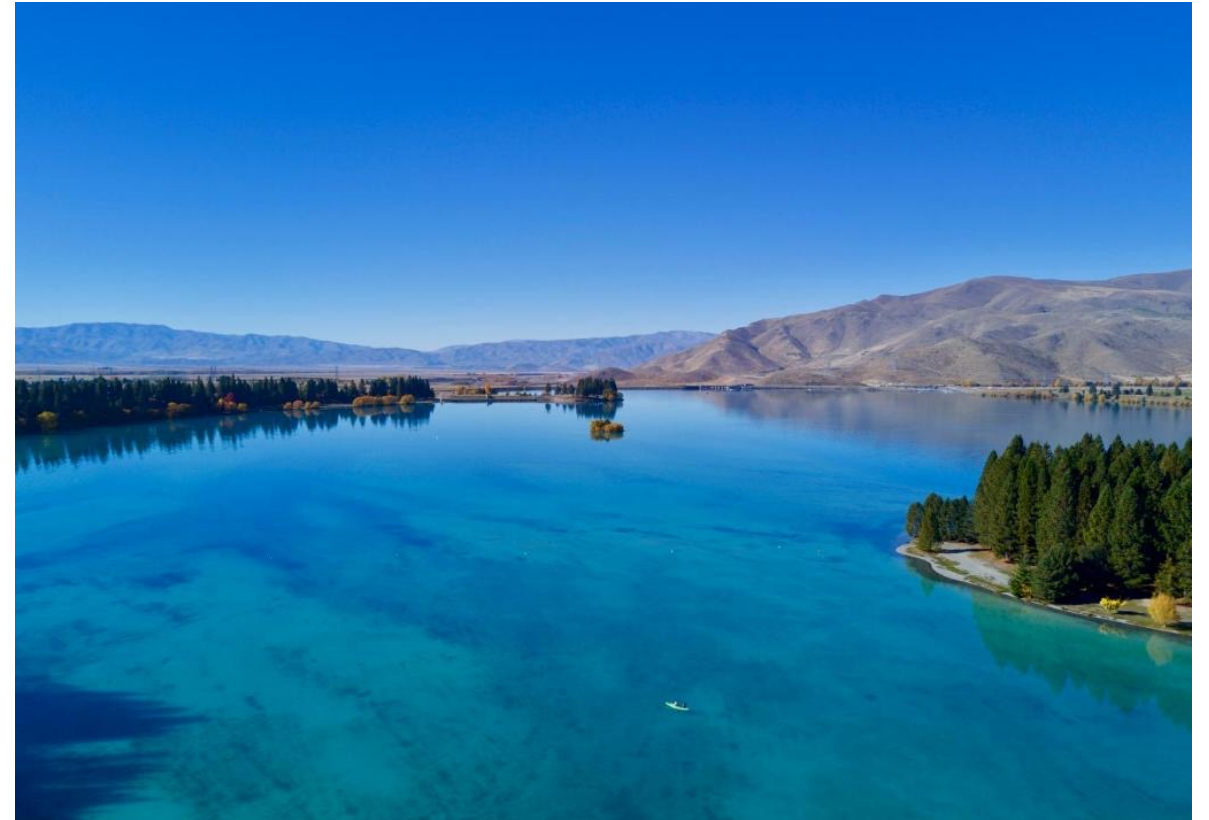
Lake Ruataniwha, near Twizel, part of Meridian's Waitaki hydro scheme
