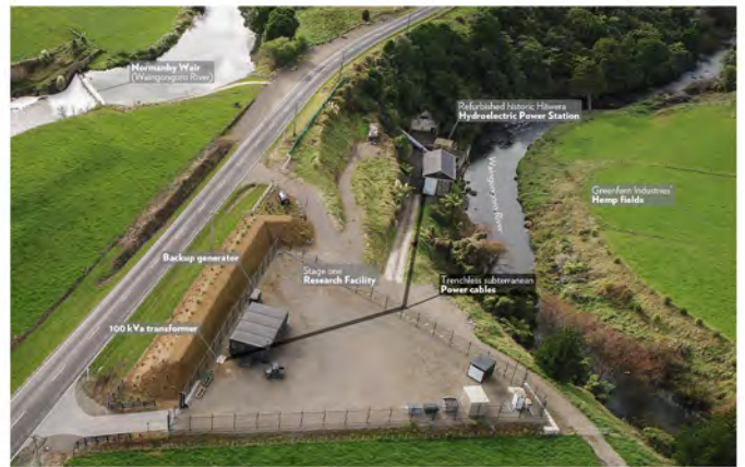
GreenFern power station and facility in Normanby Taranaki
