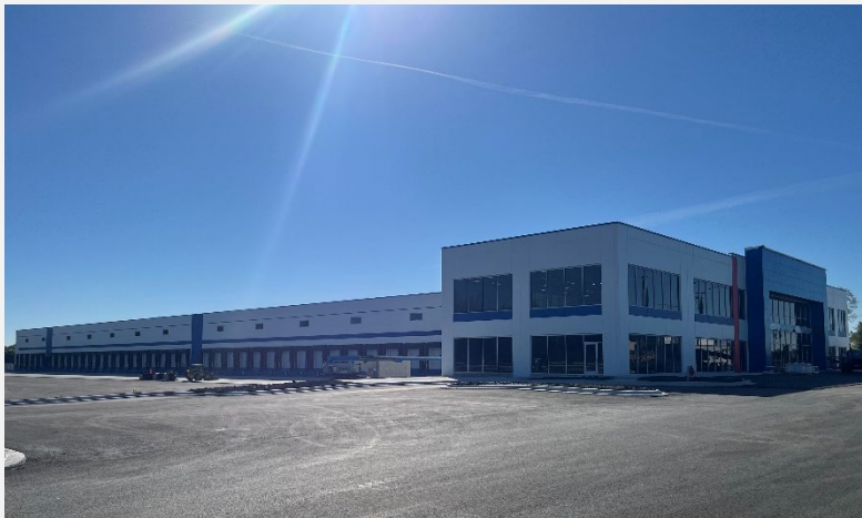
Chicago Transport Cross-dock
