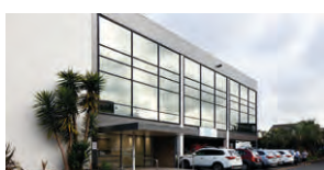
308 Great South Road, Greenlane
