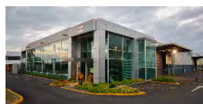
106 Springs Road, East Tamaki
