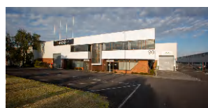
90-104 Springs Road, East Tamaki
