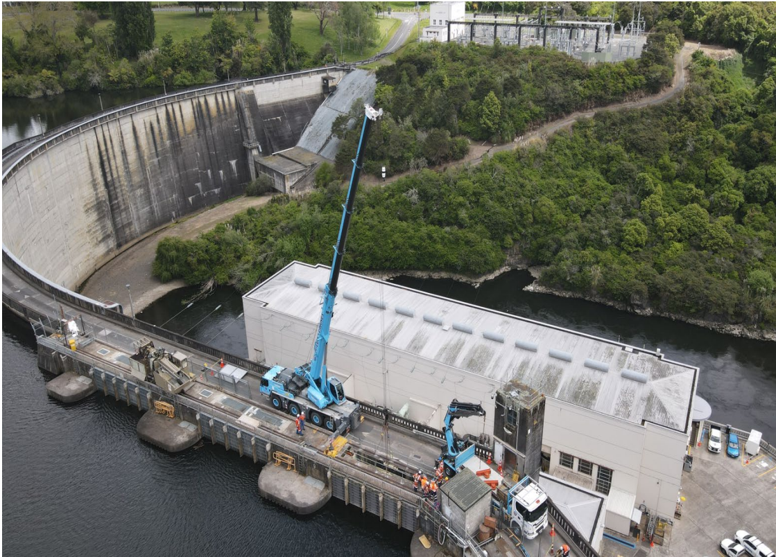
Karāpiro head gate installation
