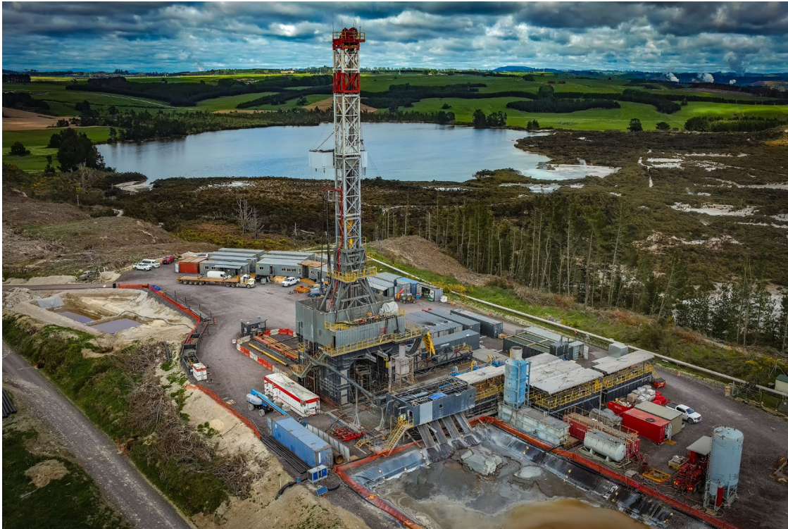
Geothermal drilling rig at Rotokawa
