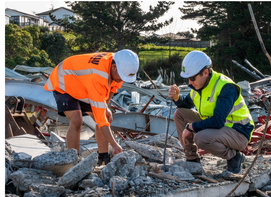
Roma Road Estate – Demolition waste diversion
