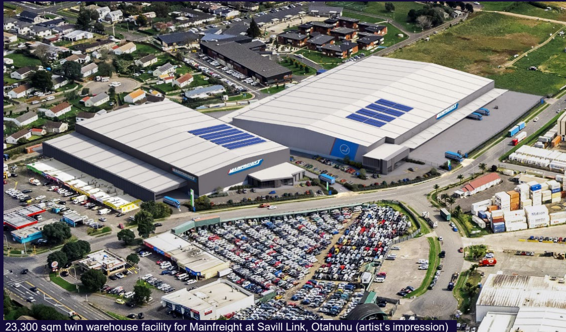
23,300 sqm twin warehouse facility for Mainfreight at Savill Link, Otahuhu (artist's impression)
