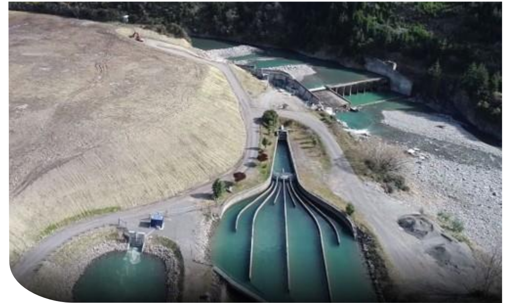
New Branch infiltration gallery with discharge into the Argyle Canal on the left
