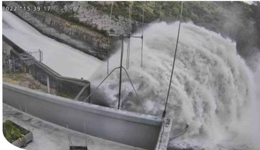
Matahina spillway at 150 cubic metres per second
