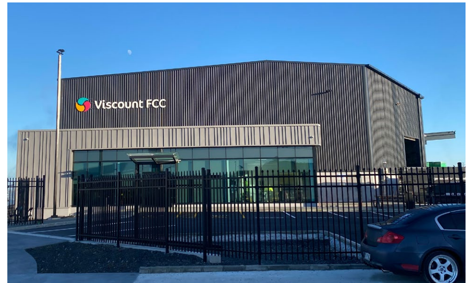
➤ The twin North Point warehouses at Highbrook Business Park completed in July 2023. They provide almost 8,000 sqm of office and warehouse space.
