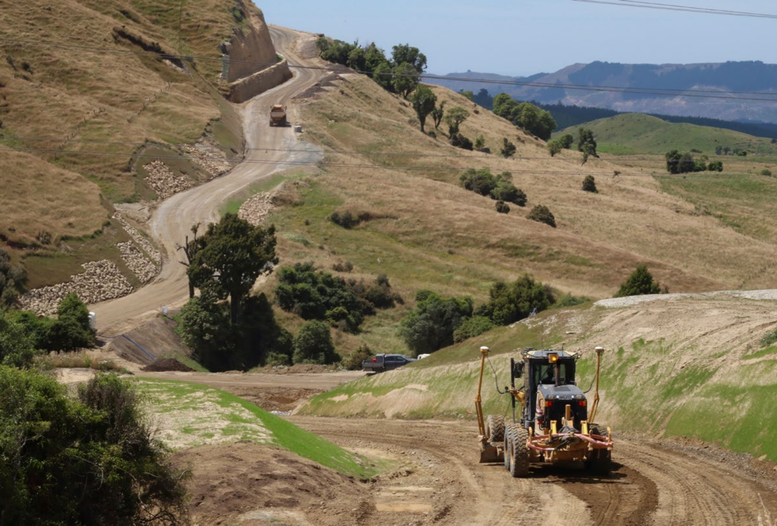
Road construction at Meridian's Harapaki wind farm, near Napier
