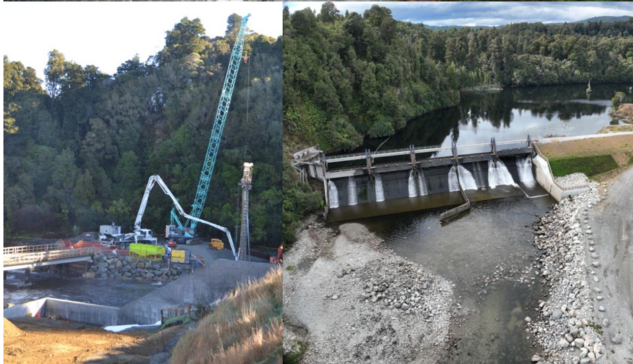
Piling works to strengthen Arnold Dam.
