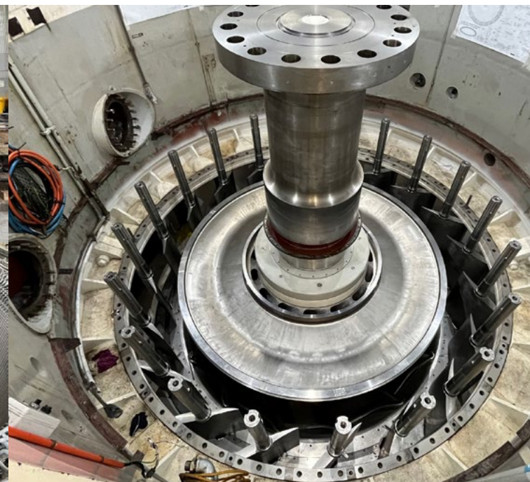
New turbine installation.
