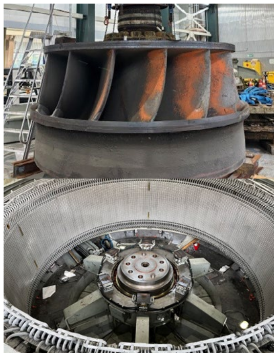
Original turbine runner being removed after 57 years of service.
