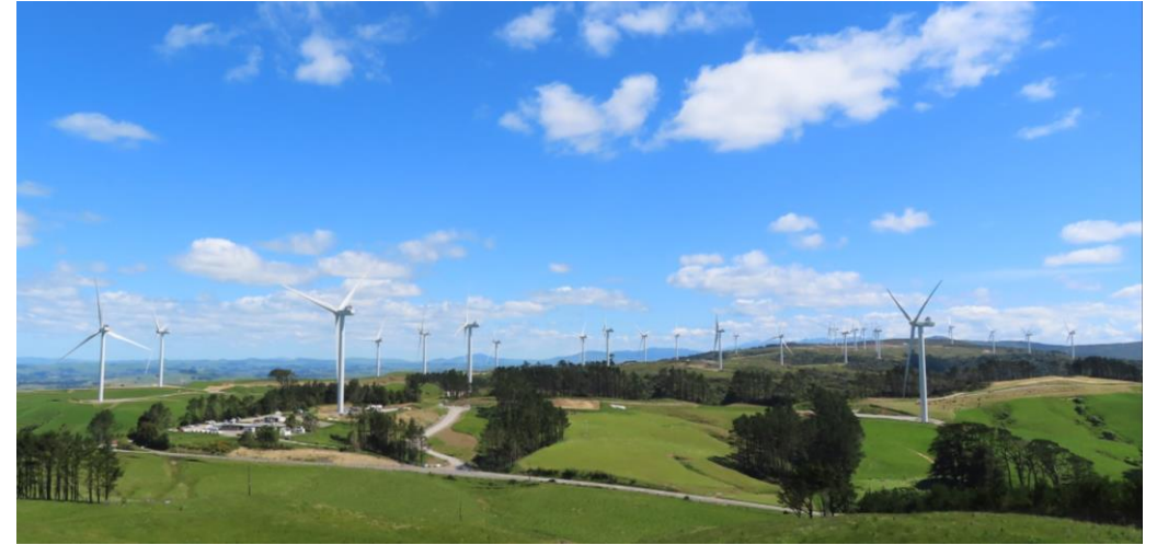
Turbines at Turitea North
