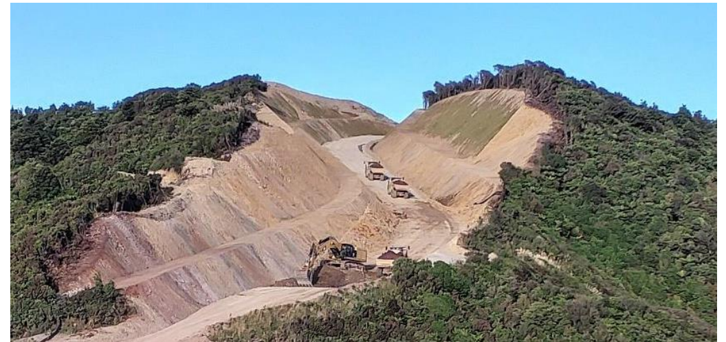
Turitea South access road construction between turbines 36 and 37
