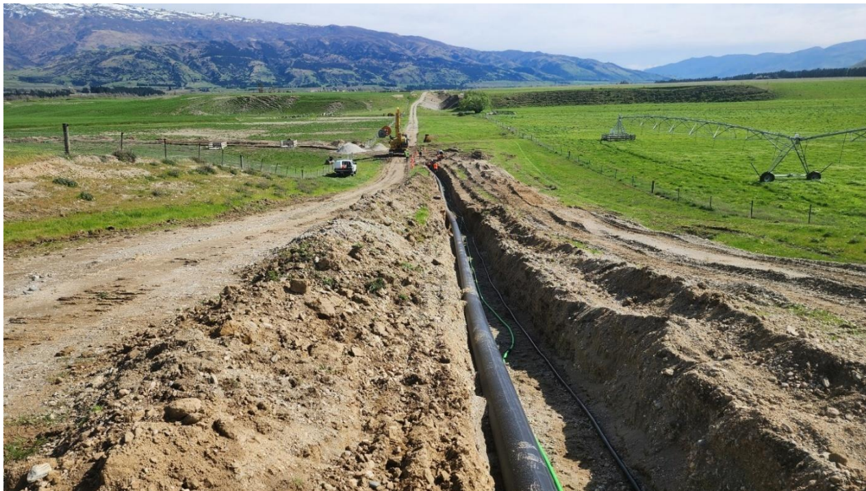
Figure 3: Permitted Early Works – Installation of 1km of Mine Water Pipeline
