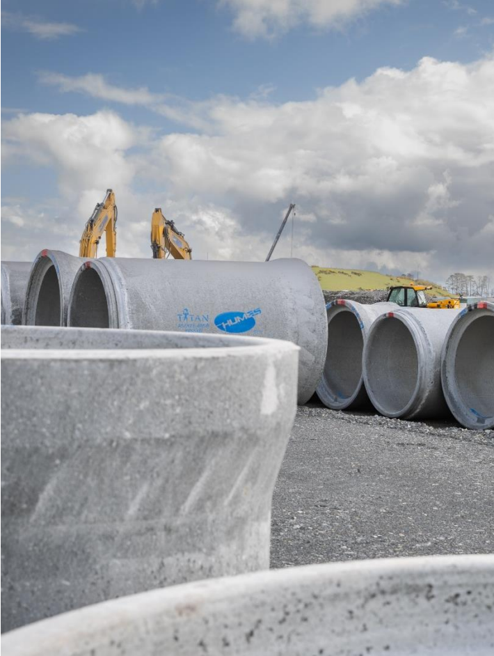
Stormwater pipes awaiting installation
