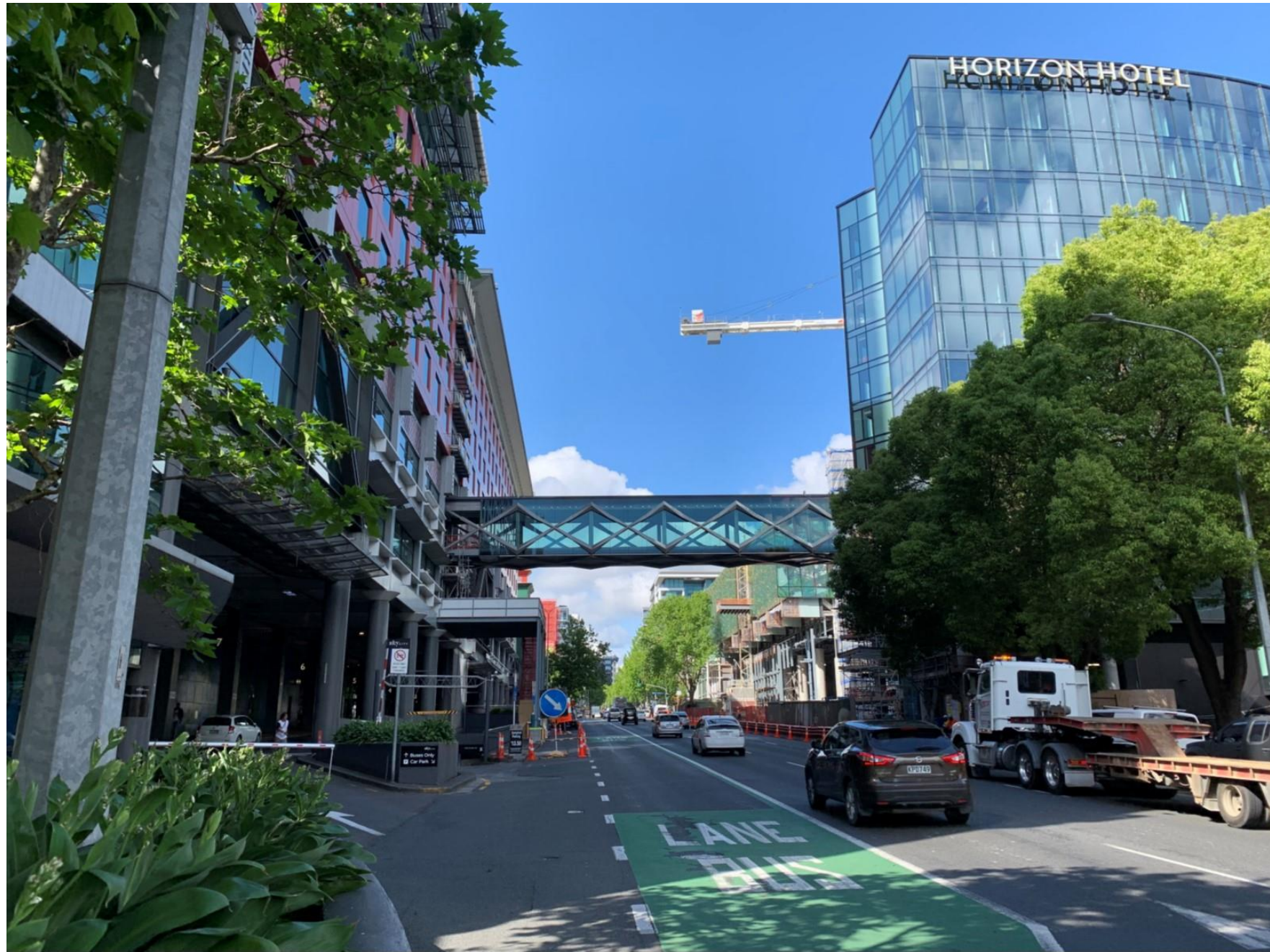
View from Hobson St – new linkway bridge
