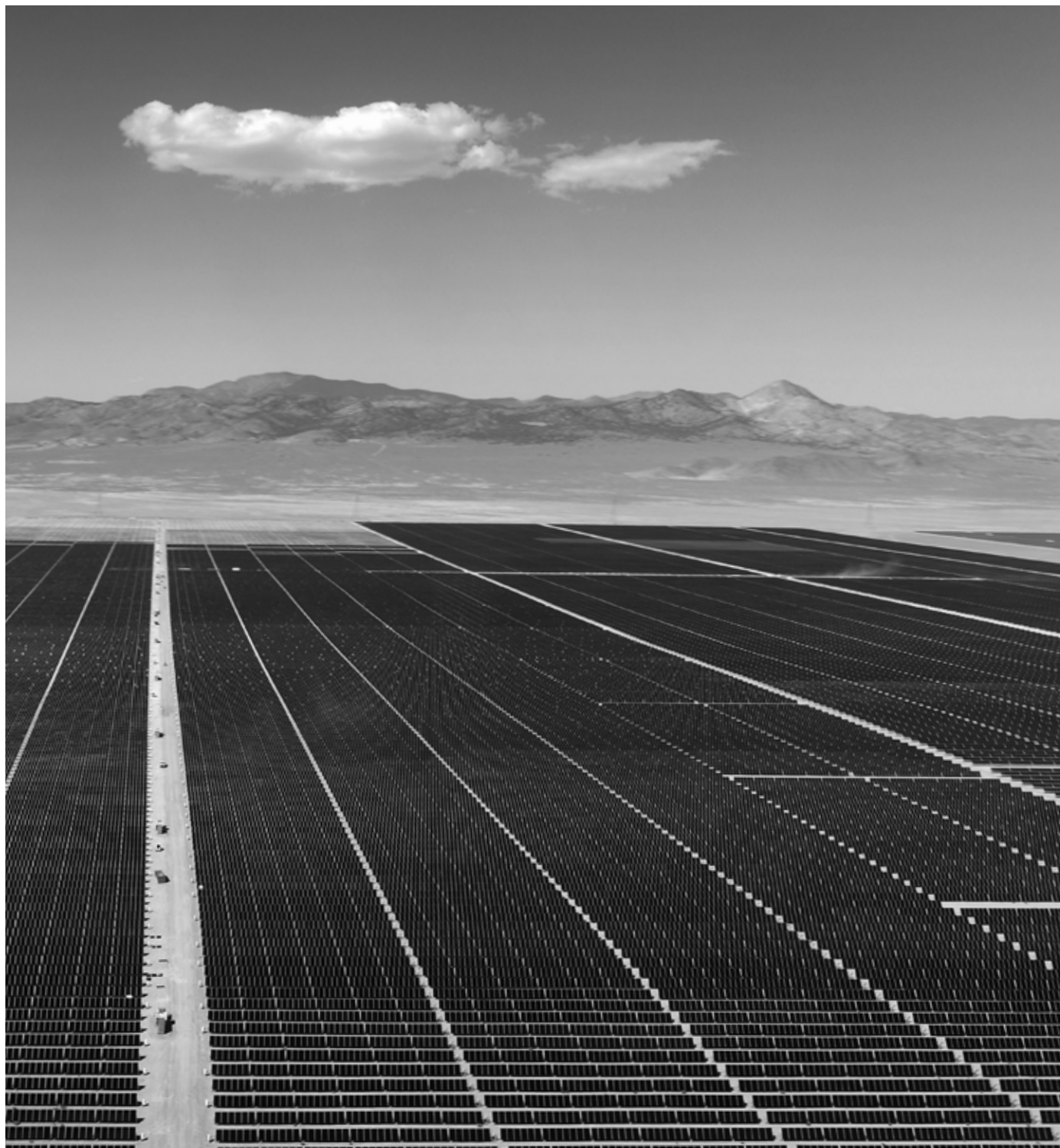
Prospero Solar project, Texas, USA.
