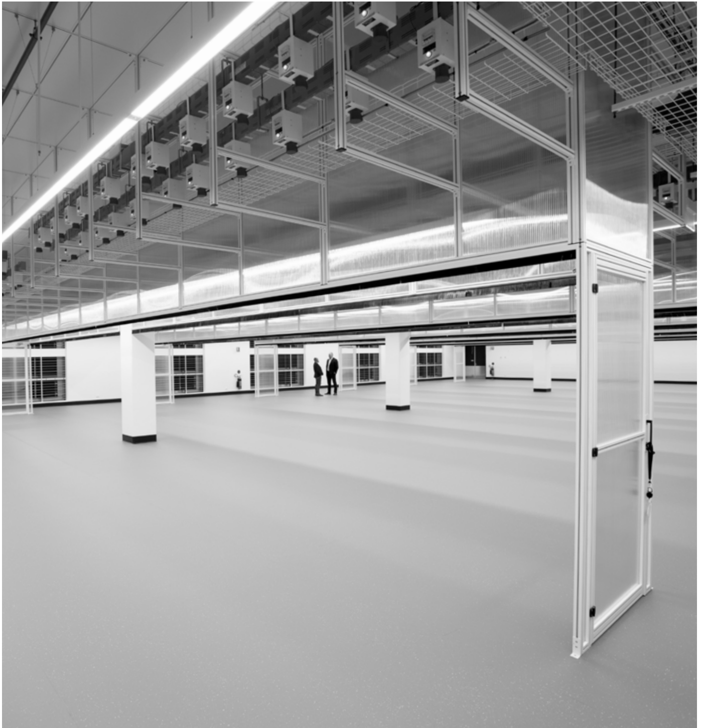
CDC data centre prior to internal fit out
