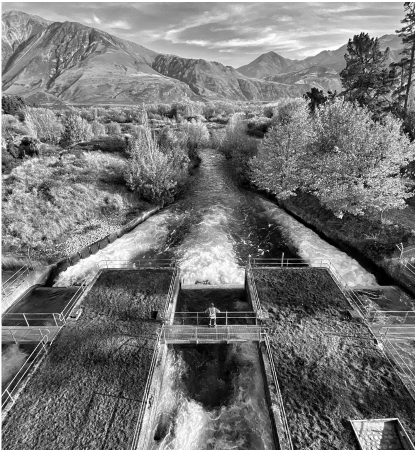
Lake Coleridge Power Station
