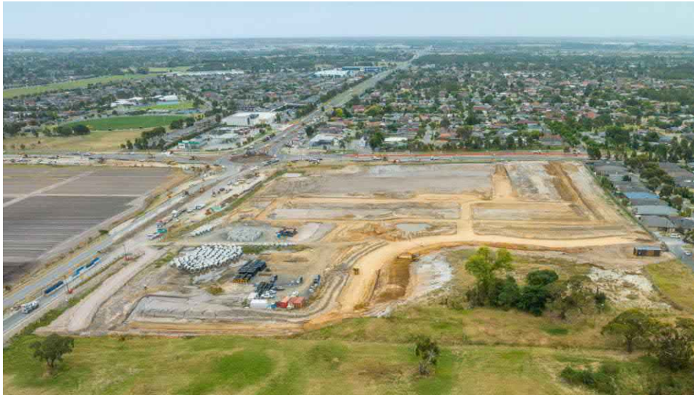
Summerset Cranbourne North (Melbourne)
