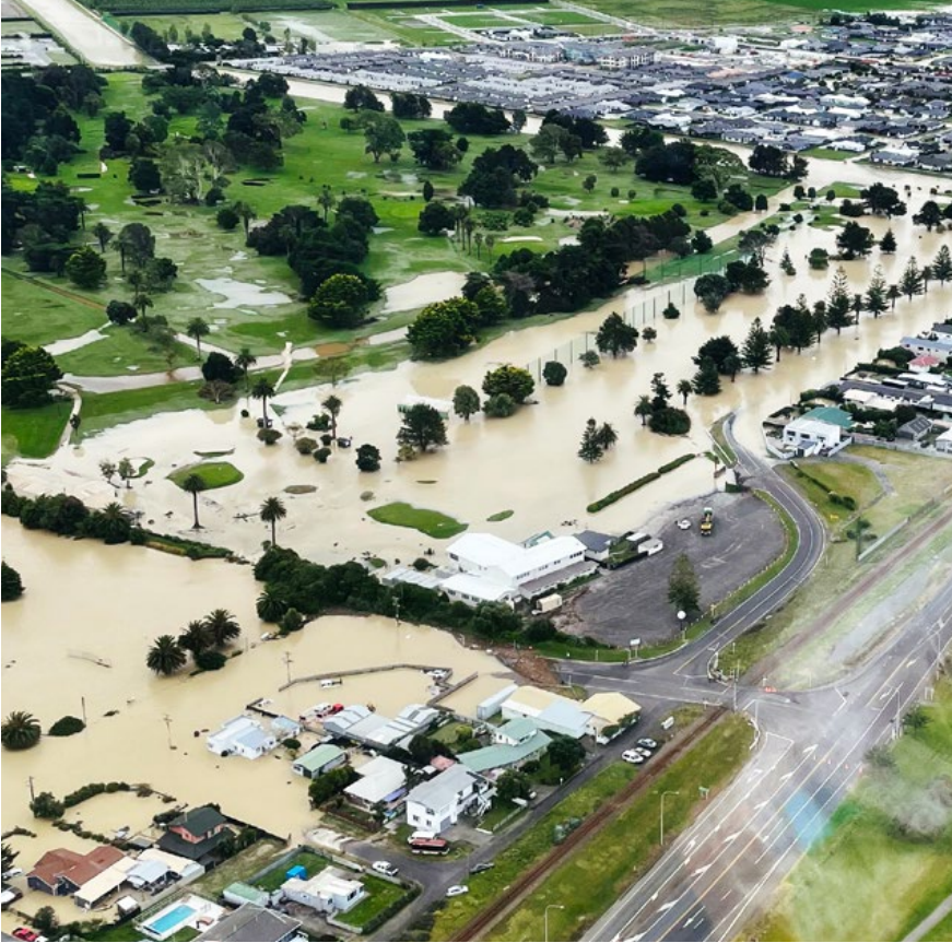
Flooding caused by Cyclone Gabrielle.
