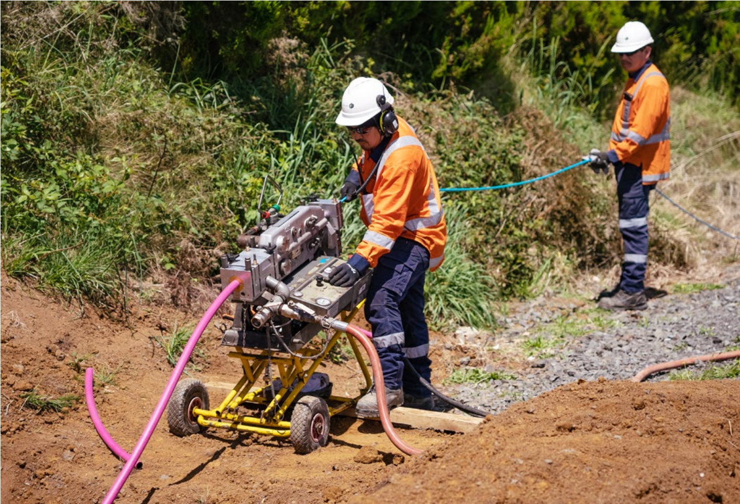
Entelar Group 1 team members completing an on site installation.
