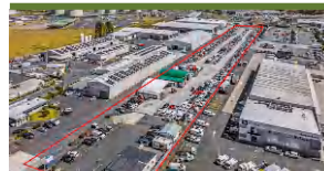
133 Roscommon Road, Wiri
