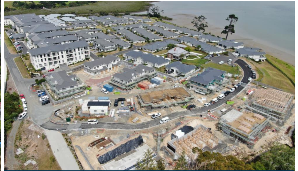
Summerset at Monterey Park (Hobsonville, Auckland)
