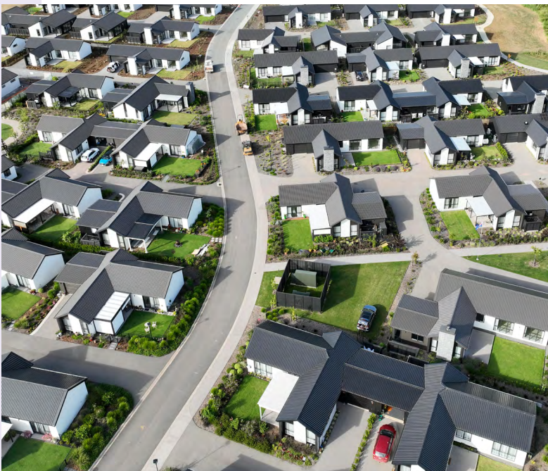
Villa development continues at Te Puna Waiora, Kerikeri
