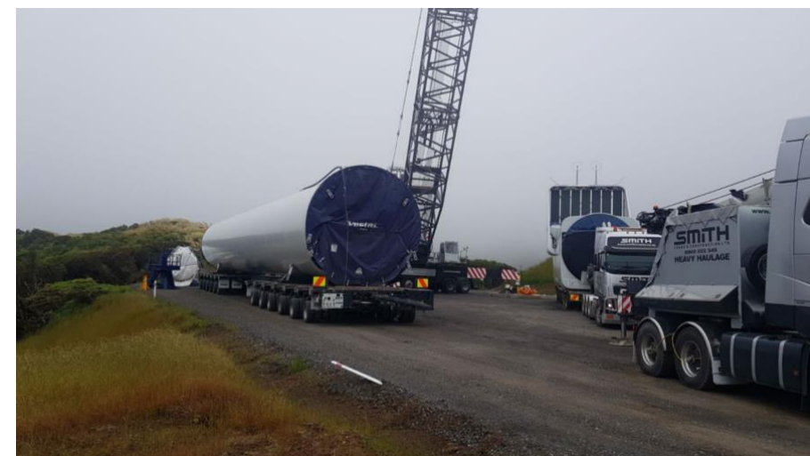
Towers being transported to site for erection
