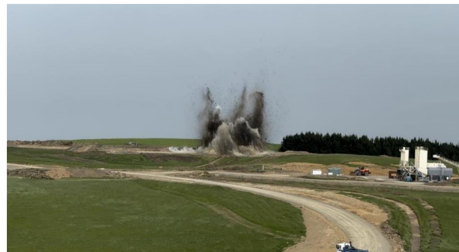
Foundation blasting at Kaiwera Downs
