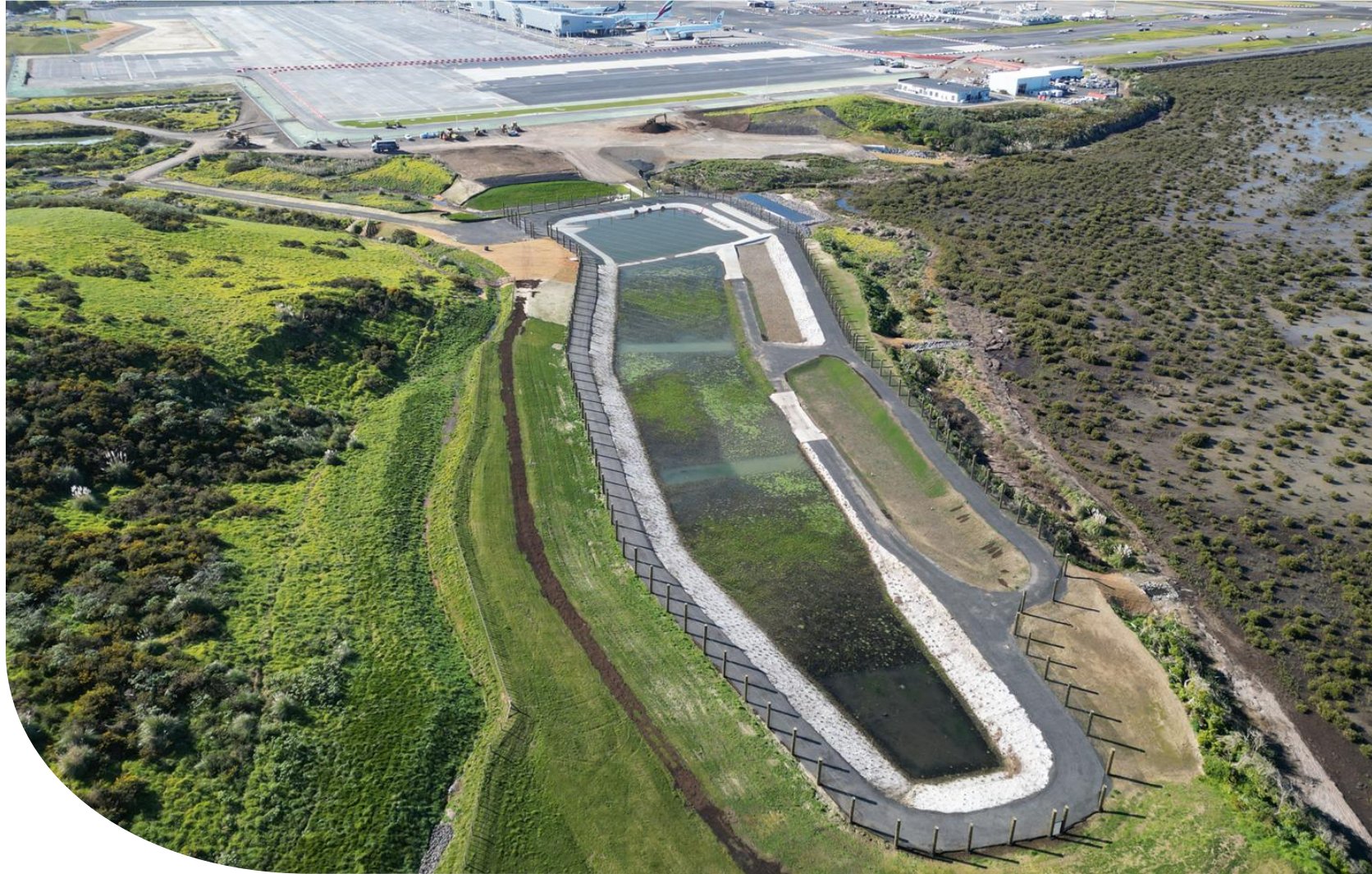
New biofilter stormwater pond
