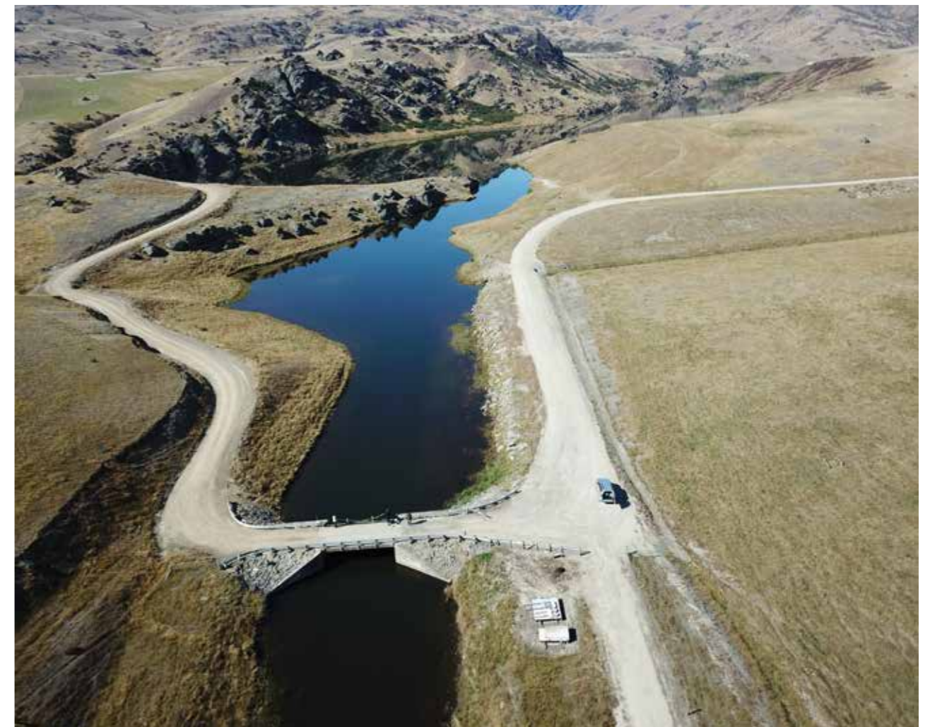
Our Paerau Canal intake.
