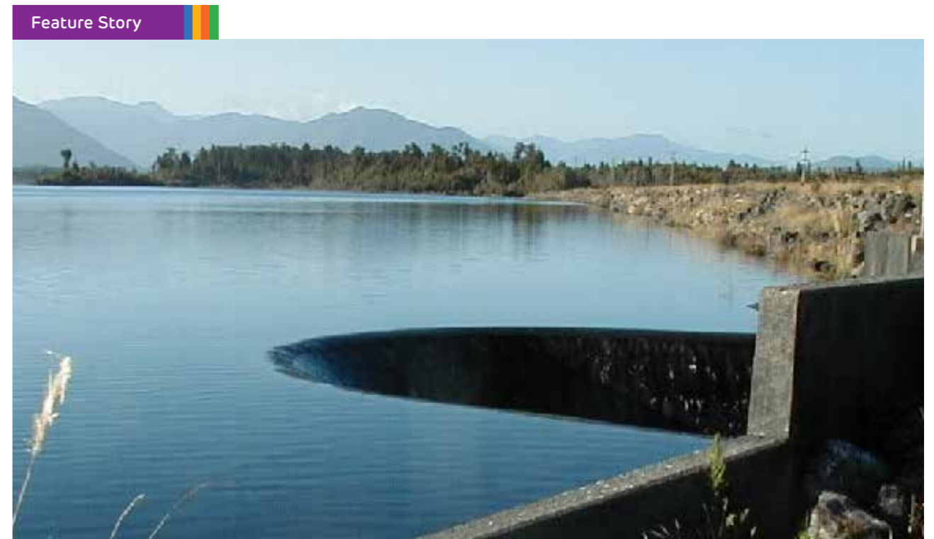
An overflow spillway at our Dillmans West Coast Hydroelectric Power Scheme.
