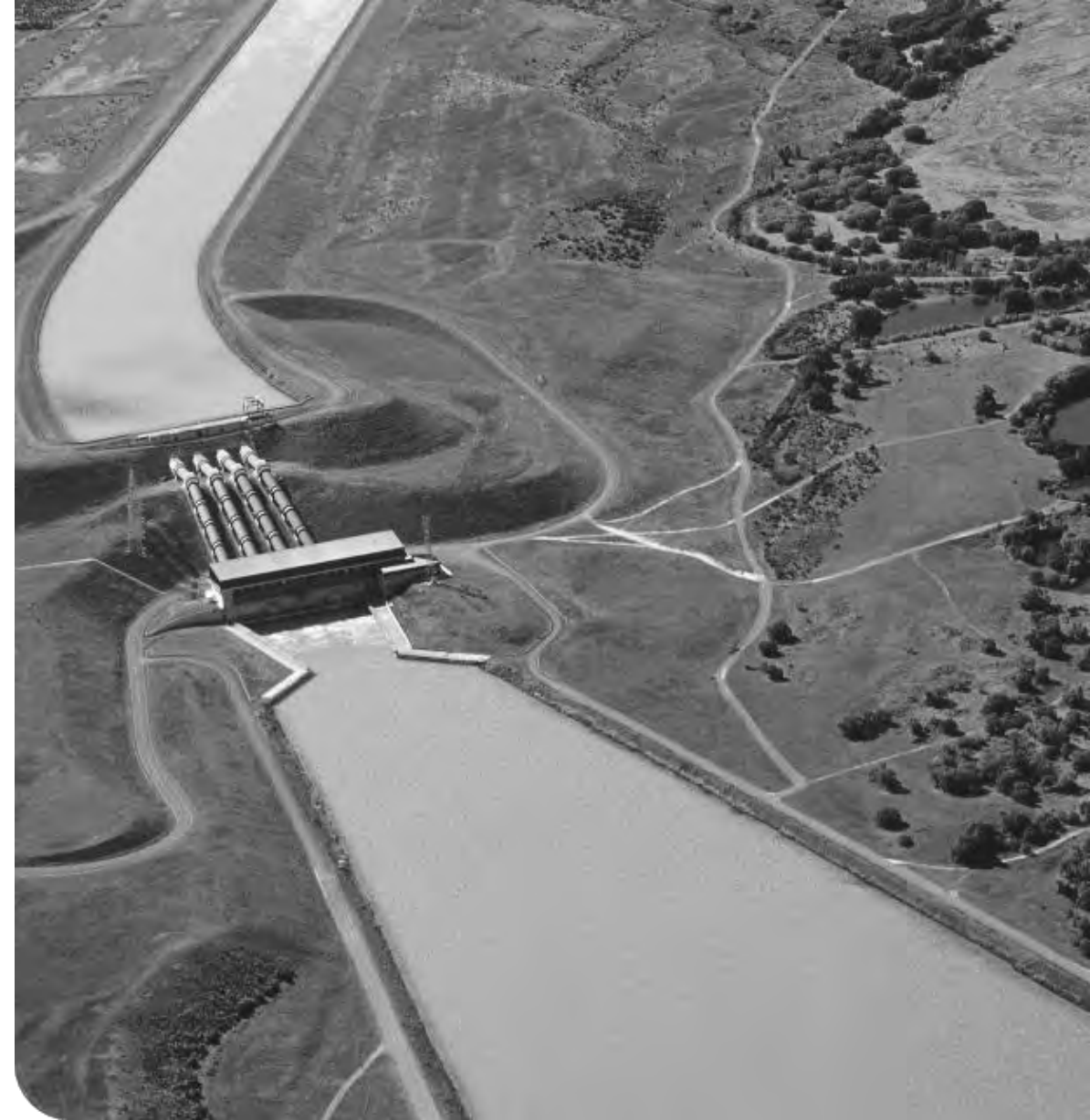
Ōhau C Power Station.
