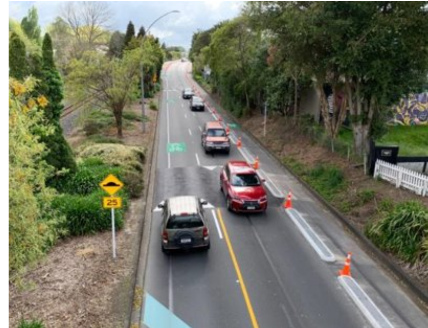
Hamilton Infrastructure Alliance
