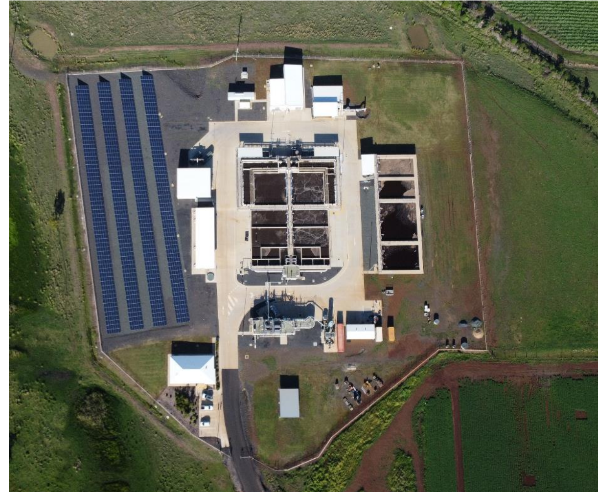
Rubyanna wastewater treatment plant
