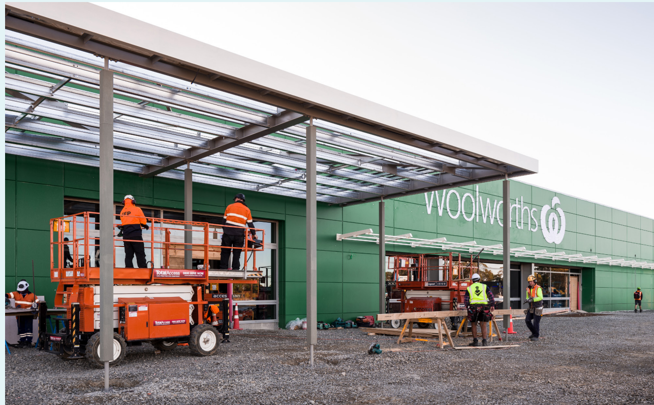
Woolworths in development, Waimakariri Junction
