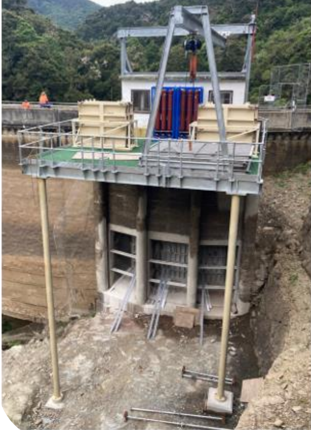
Upgrading intake structure for 4 station
