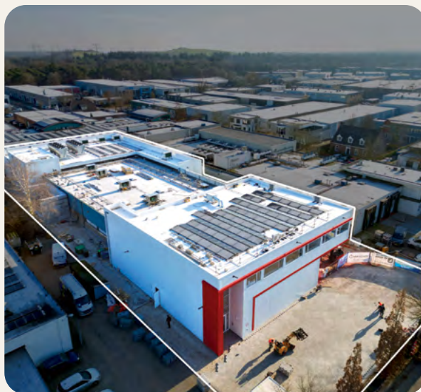
New processing facility under construction in the Netherlands
