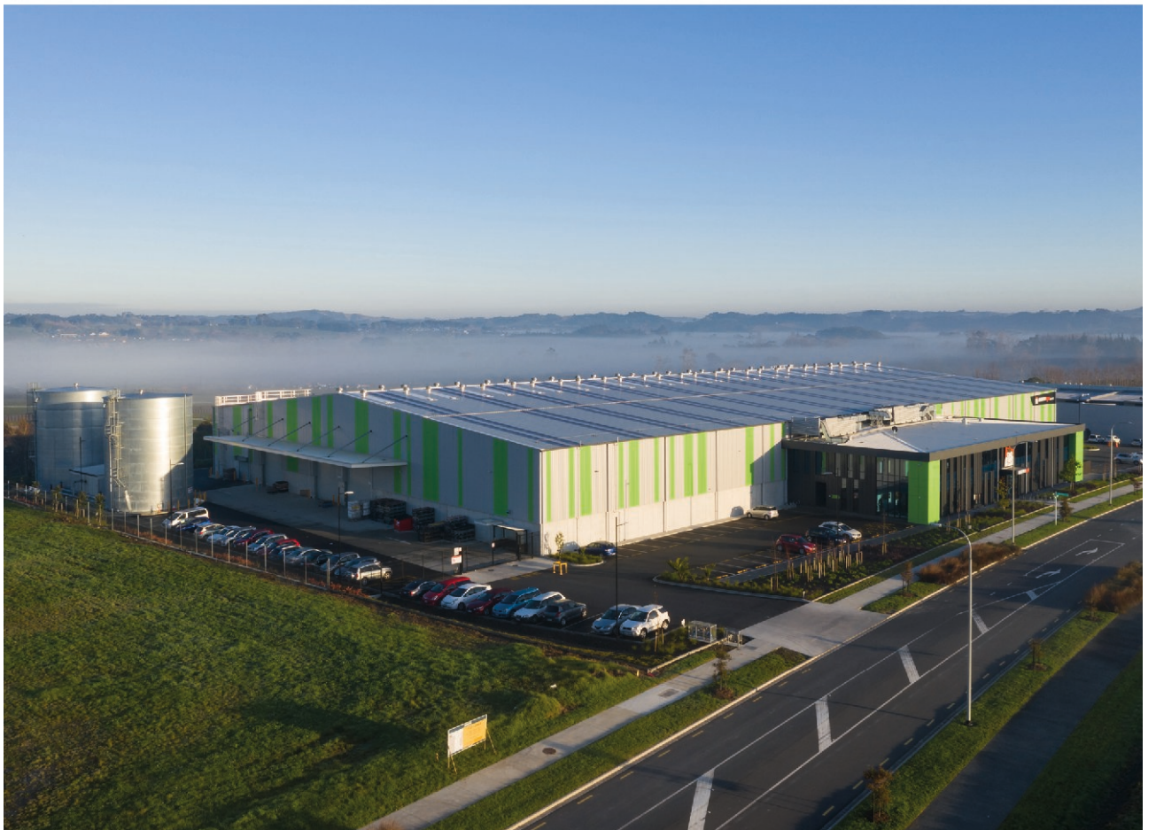
Top: 107 Carlton Gore Road, Auckland. Bottom: Highgate Parkway, Silverdale.
