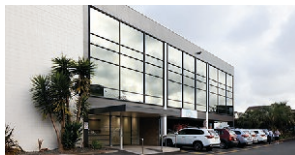
308 Great South Road, Greenlane
