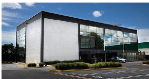
302 Great South Road, Greenlane
