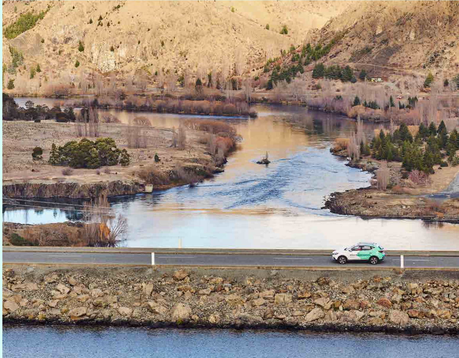
Benmore Hydro Power Station, Otematata.
